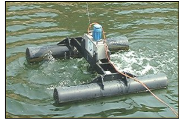
Alpha Taxiway Aeration Pond
